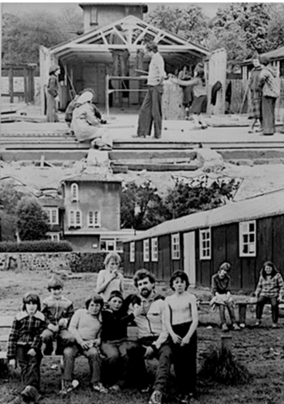
Construction of HYPs Bothen Adventure Playground 1971. Then project worker and now CEO of Sporting Communities Kevin Sountry seen sitting with young people
